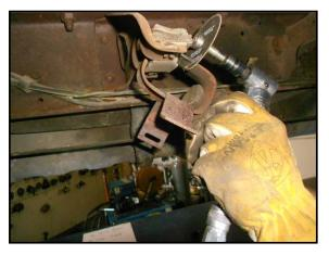
Remove the factory pipe hangers from the front and middle exhaust hanger mounts.
